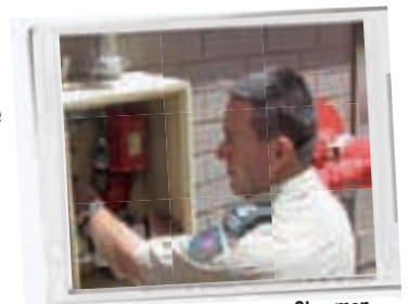
Training Officer Darren Chapman commissions a Domestic Sprinkler System, recently installed into the multi-storey building at the CFS State Training Centre.
